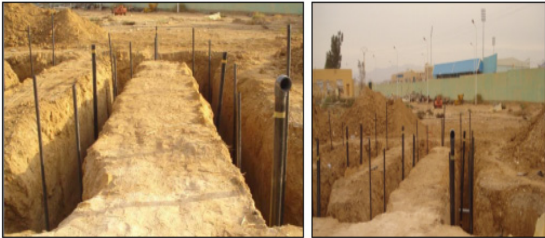
Fig. 1. Trenches for installation of the buried air / ground heat exchanger [23]
